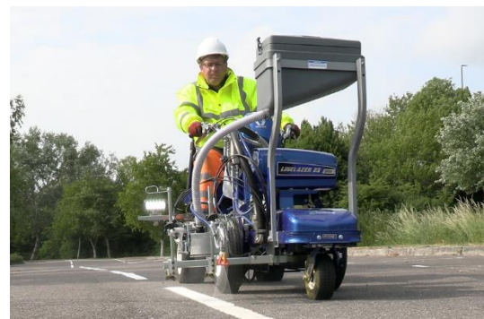
Cold applied line marking system
