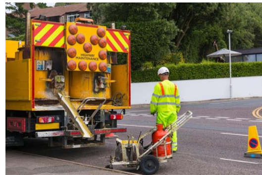
Thermoplastic applied linemarking systems
