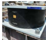
Lead Rubber Bearing (LRB)
