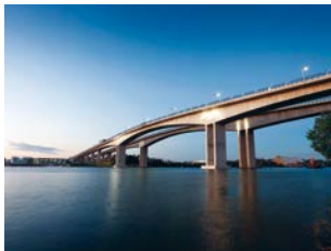
Gateway Bridge, Australia
