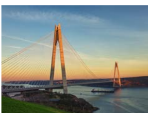
Third Bosphorus bridge, Turkey
