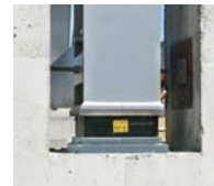
Reinforced elastomeric bearing
