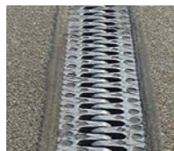
Cantilever finger joint
