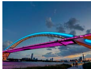
Lupu Bridge, China
