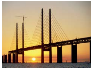
Öresund Bridge, Denmark
