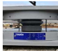
Pendulum bearing
