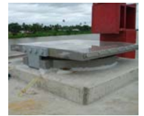
Incremental launch (ILM) bearing
