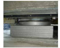
Spherical bearing
