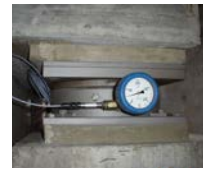
Lifting and measuring bearing
