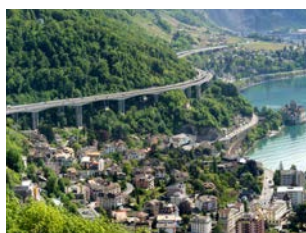
Viaduct de Chillon, Switzerland
