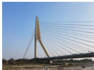
Wazirabad Bridge, India
