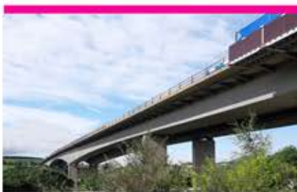
FRIARTON BRIDGE Perth, Scotland
