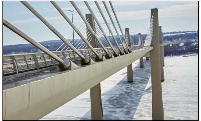
St. Croix River Crossing
