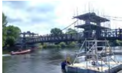
Our award-winning restoration design work on the 1889 Ferry Bridge at Burton-on-Trent.
