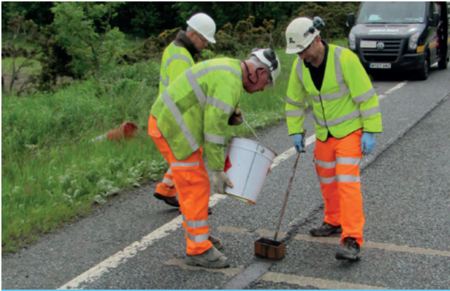
SAFETRACK® INLAID ROAD REPAIR APPLICATION
