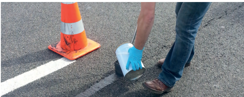
SAFETRACK® CRACK INFILL APPLICATION
