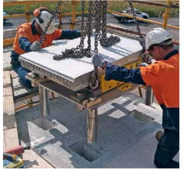
Gerringong Bridge Australia
