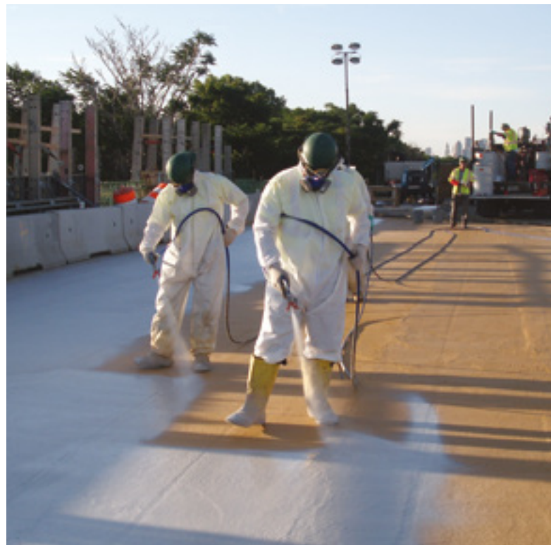
APPLYING SECOND COAT OF ELIMINATOR®
