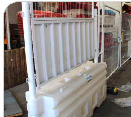
Half hoarding & fence next to vehicle gate
