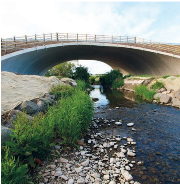
Bridge Over Water
