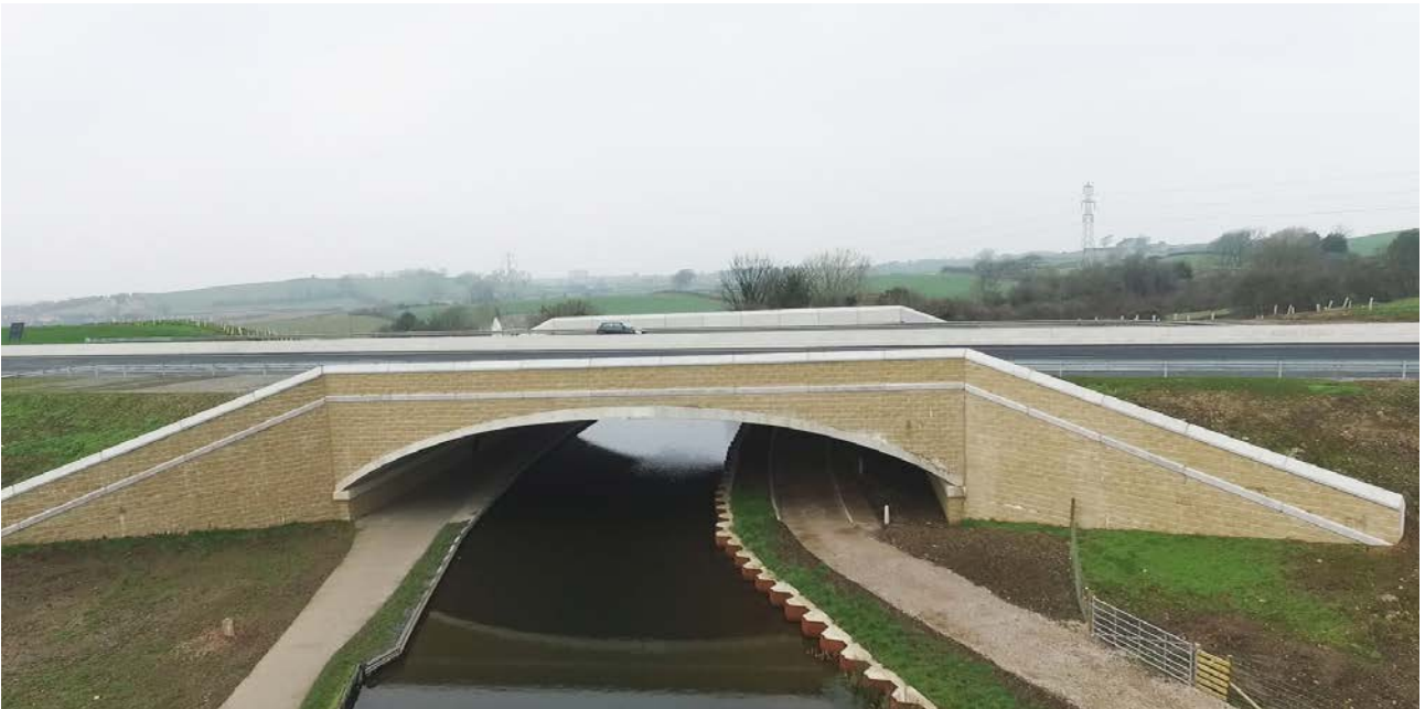
Heysham to M6 Link - Milestone Canal Bridge(654BI) (asset BEBO® Arch T94S - Span 28.651m - Rise 3.213m)
