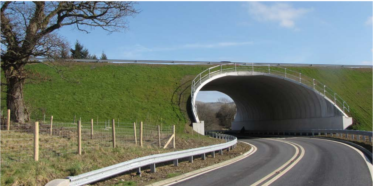
A470 Cwmbach to Newbridge -on-Wye- Red House Bridge (asset BEBO® Arch E15.5Mt/5 - Span 15.5m - Rise 5.6m)
