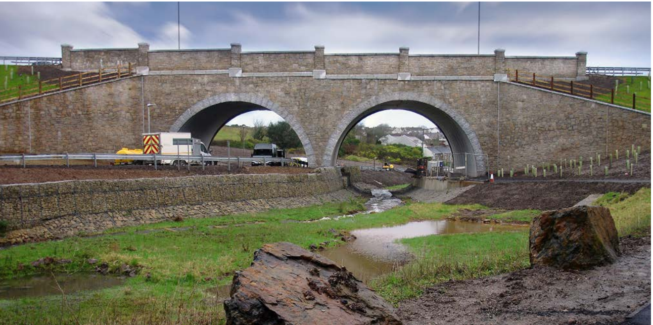
Camborne Pool - Redruth East - West Link - Red River Valley Arches (asset BEBO® Twin Arches C42T/5 - Span 12.802m - Rise 6.807m)
