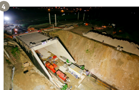
4 - Final sliding and backfilling
