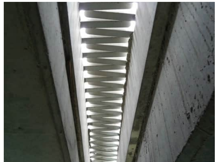
WP joint seen from below
