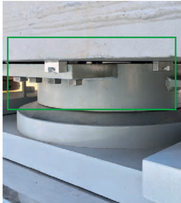
Gap compensation at bridge bearing, Yavuz Sultan Selim Bridge, Istanbul, Turkiye
