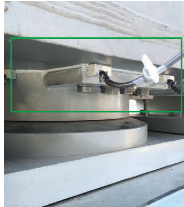
Gap compensation at bridge bearing, Yavuz Sultan Selim Bridge, Istanbul, Turkiye
