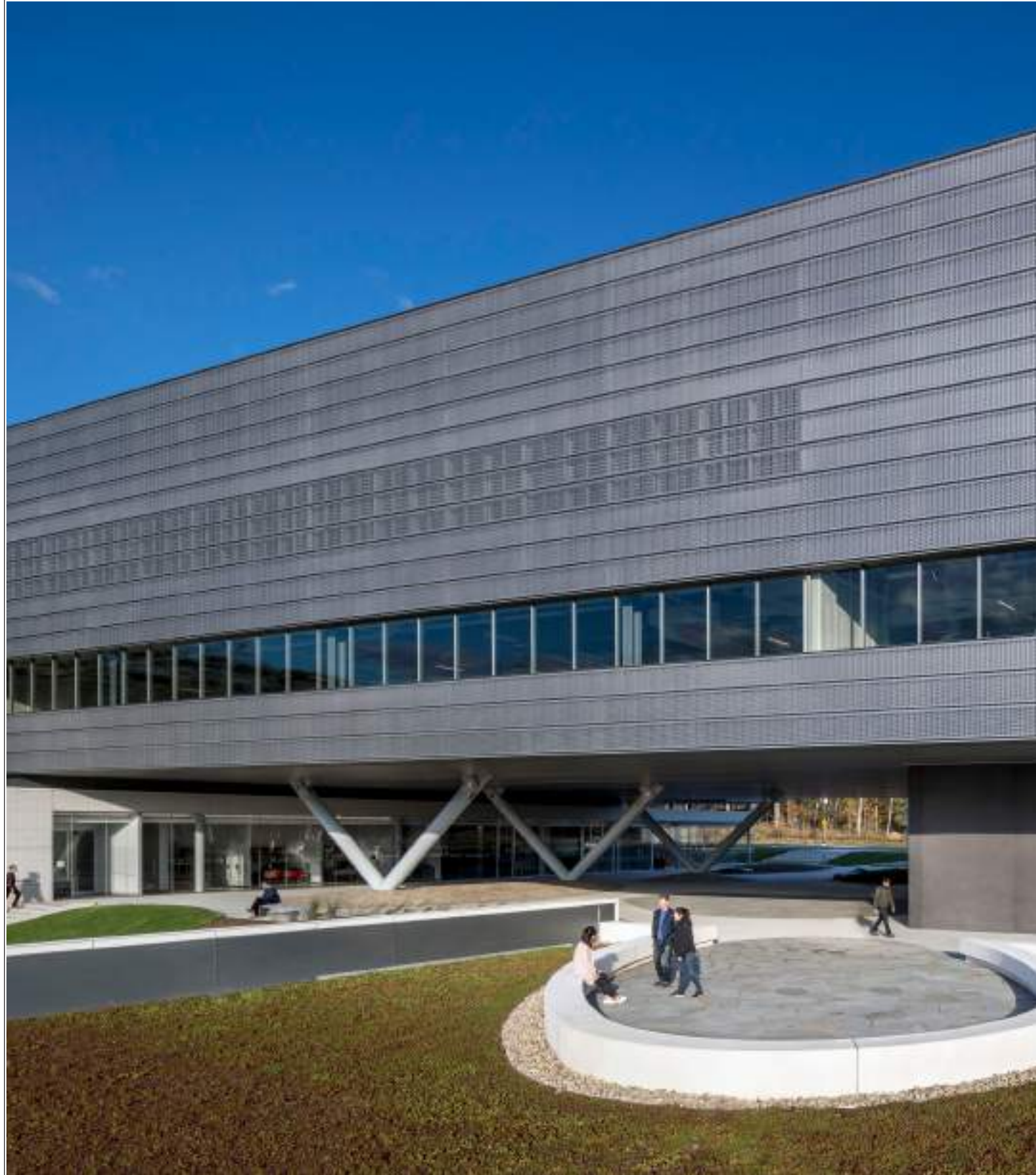
University of Connecticut Innovation Partnership Building Storrs, CT
