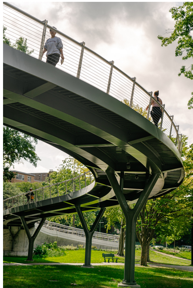
Figure 7: The Frances Appleton Pedestrian Bridge, completed in 2019, features cast steel nodes at the intersections of the HSS-12.75 branch members and the built-up trunk of bridge piers.
