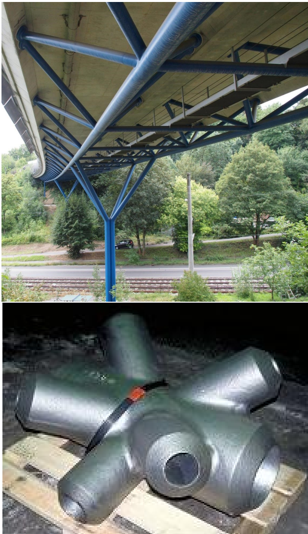
Figure 1: Use of round hollow sections and cast steel nodes enables the vehicular bridge (above) to achieve structural performance criteria with minimal tonnage and lightness in form. The custom cast steel node (directly above) sits at the
