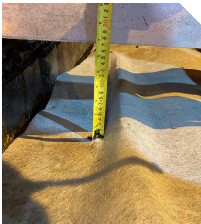
Using the IKO PermaFLASH D300, we plugged the air gap and then applied a primer to all trench surfaces. After the primer came a first layer of molten PSB, which is a highly flexible material used for tanking the trench. It was applied to the base of the trench, and a galvanised steel plate was placed in the trench. The trench could then be fully tanked out and we installed a drainage channel and rodding box.
