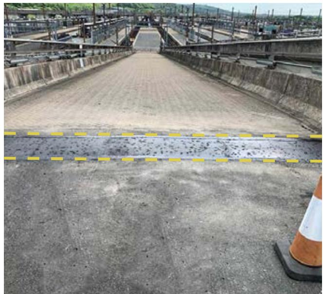
IKO provide Metrail with product and technical support as required. The IKO Permatrack H heavy duty joint is a structurally enhanced movement joint ideal for repairing and replacing damaged joints and able to accommodate the movement inherent in bridges and decks.
