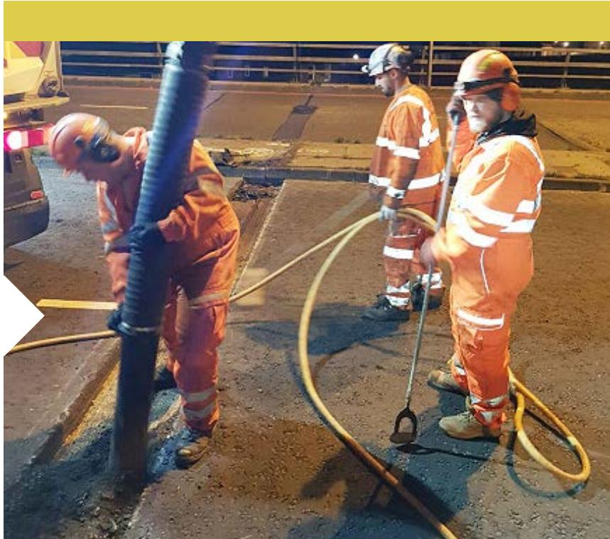
**The joint material caters for +/- 20mm movement range (40mm total)**
