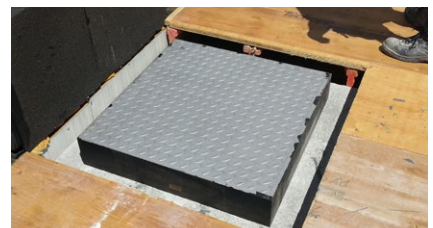
Example of a LASTO®BLOCK deformation bearing with chequer plate
