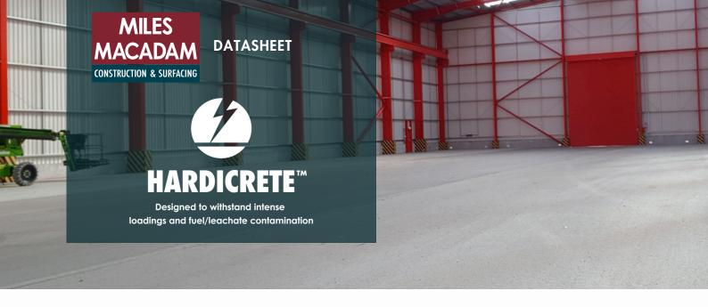
Hardicrete™ is a BBA certified (Agrément Certificate Number 88/1969) Grouted Macadam surface course designed to withstand intense traffic loadings and fuel / leachate contamination. The company is certified to National Highways Sector Scheme 16 for Quality Management in Highways Works.
