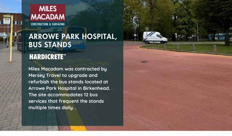
The existing material had suffered deformation and rutting due to heavy traffic and constant bus movements. The project also involved reprofiling the drainage system and gulleys to enhance drainage and surface water retention.
