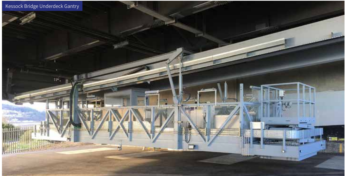
Kessock Bridge Underdeck Gantry
