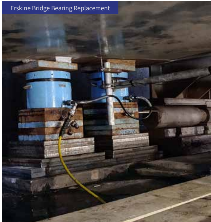
Erskine Bridge Bearing Replacement
