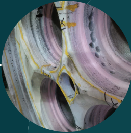
Fractures due to overheating or third-party arc welding
