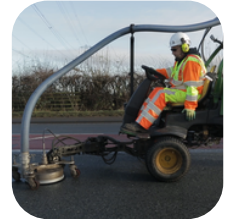
Hydroblast Removal
